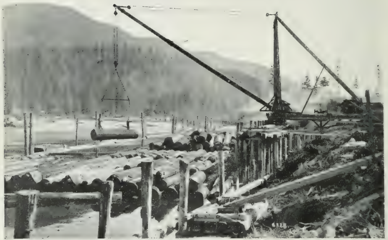
FIG. 100. BUILDING SEA-GOING LOG RAFT: BRITISH COLUMBIA. [By courtesy of Canadian Government.]
